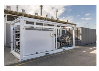
Dresden/USA, 29.02.2016. sunfire has developed the world's largest commercial reversible electrolysis (RSOC) module and delivered it to U.S. partner Boeing. The energy system uses hydrogen as its storage medium and ensures the reliable supply of electricity originally generated using wind power or photovoltaic arrays. It is now in operation at a U.S. Navy microgrid test facility in California. The solution enables the efficient, long-term
